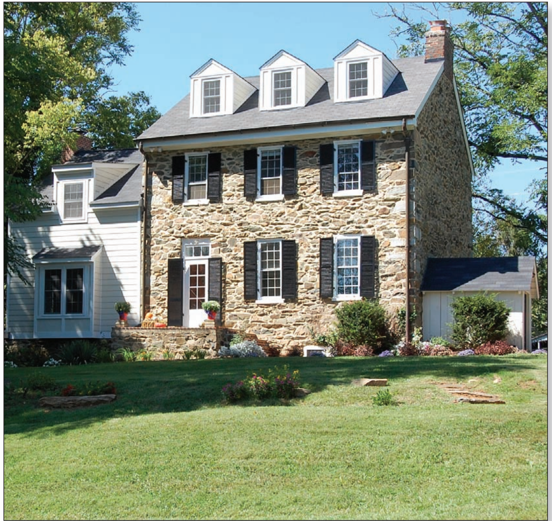
This 19th century stone home has been carefully restored using The Department of Interior Guidelines wherever possible.
